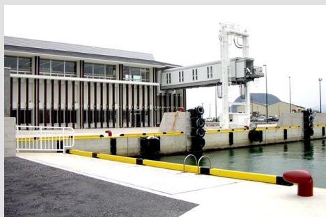
角型鋼管車止め
